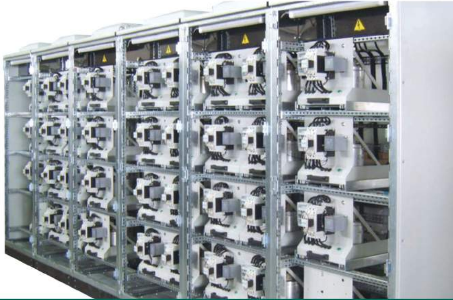
Mardin Cement Factory 1475 kVAR Compensation with Drawer
