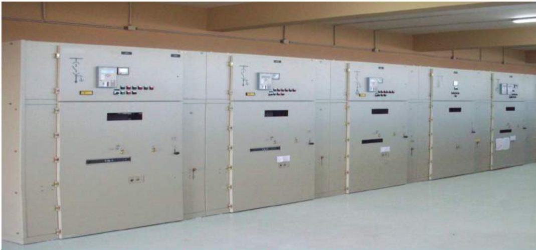
36 KV Medium Voltage Metal Enclosed Modular Switchgear
