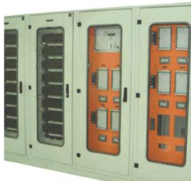
TEIAS – Kiziltepe Substation Busbar Protection Panels
