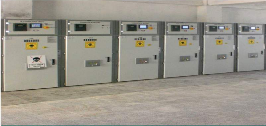
6.3 KV Medium Voltage Metal Enclosed Modular Switchgear
