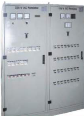
TEIAS – Adiyaman Substation AC-DC Auxiliary Service Panels (YSP)
