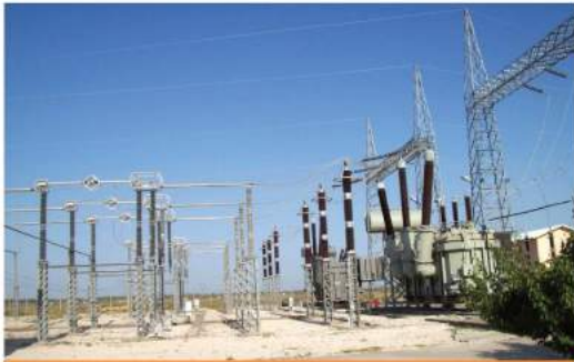
Transformers and Switchyard
