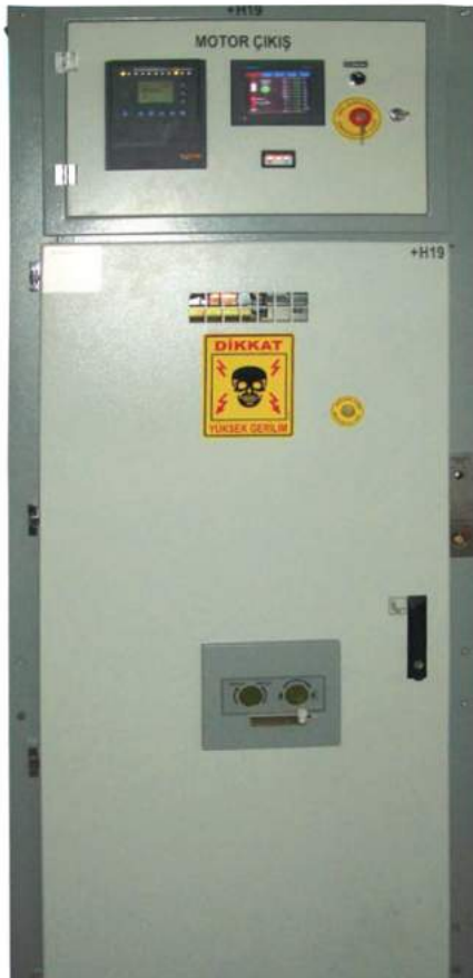
12 kV Metal Clad Cell STM-MC 12
