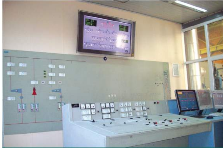
Piano type control panel
