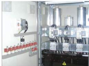
CIMSA – Eskişehir Cement Factory 1200 kVAR LV Capacitor System with Harmonic Filter
