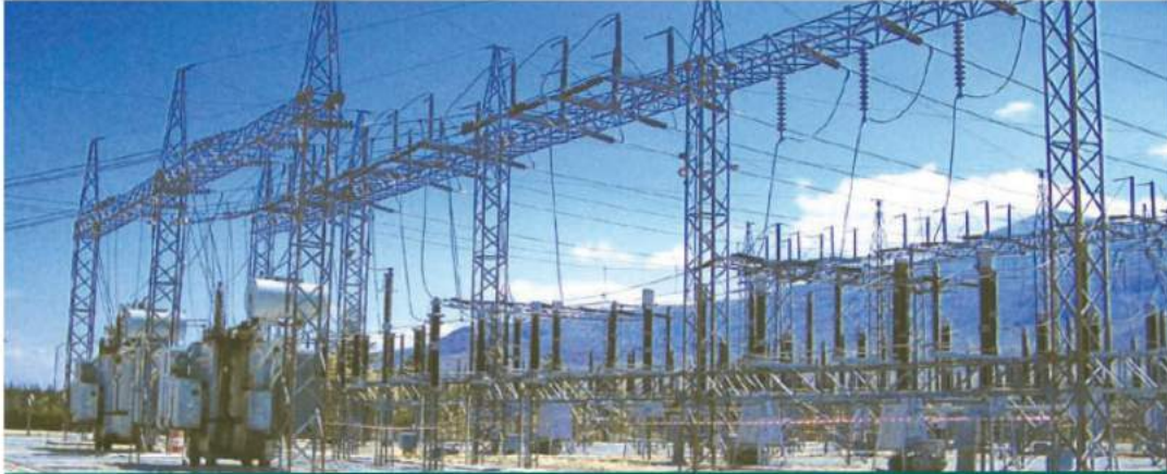
154 / 34.5 kV Switchyard System Application
