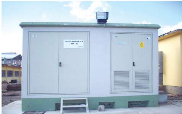
MV/LV Prefabricated Concrete Housing Transformer Substations
