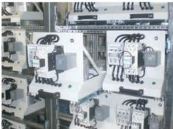
CIMSA – Eskişehir Cement Factory 1200 kVAR LV Capacitor System with Harmonic Filter
