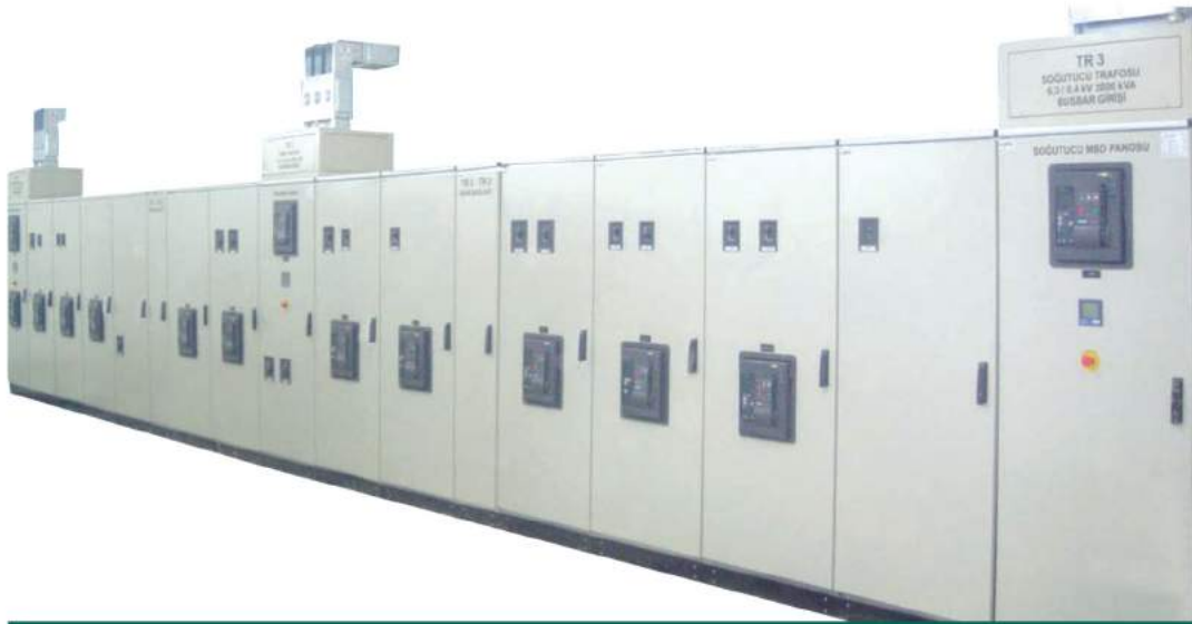
CIMSA – Eskisehir Cement Factory LV Distribution Panels and Busbar System
