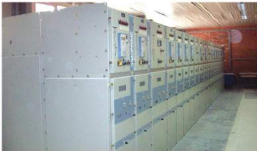
6.3 KV Metal Clad Switchgears
