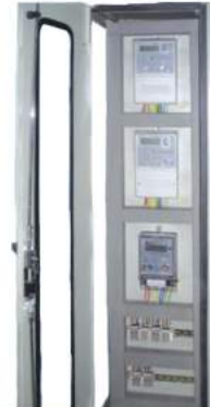
TEIAS – Tokat Artova Substation Meter Panels
